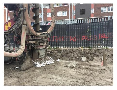
Secant Piling Works Progressing along Dominick St. Lower Elevation
