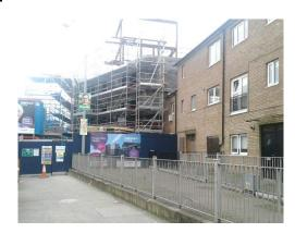
The construction of external brick/block walls is nearing completion, as are the internal stairs. The current estimated date for completion is October 2019. The finished complex will provide 29 homes for senior citizens.
